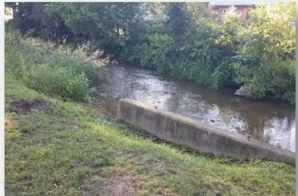
Photo 2: Loss of wall support and backfill from creek washout
