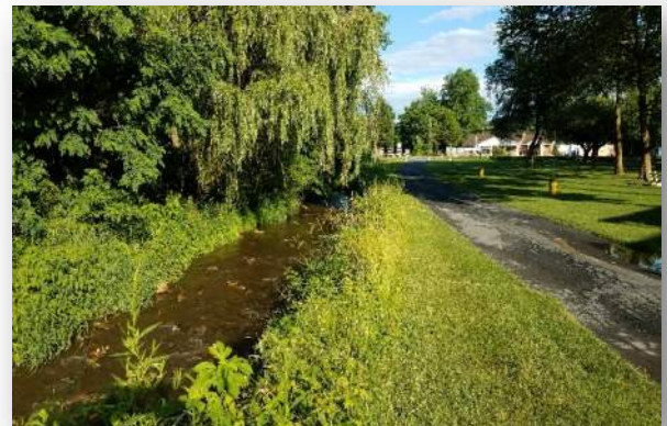
Photo 4: View of Willow Creek towards Main Street. Width of lawn area between creek and pathway has been reduced due to loss of embankment soils from erosion
