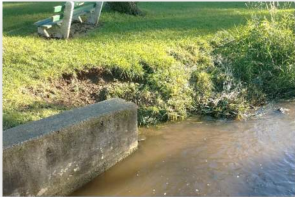
Photo 1: Area of embankment collapsing due to erosion factors from fluctuating water levels of the creek
